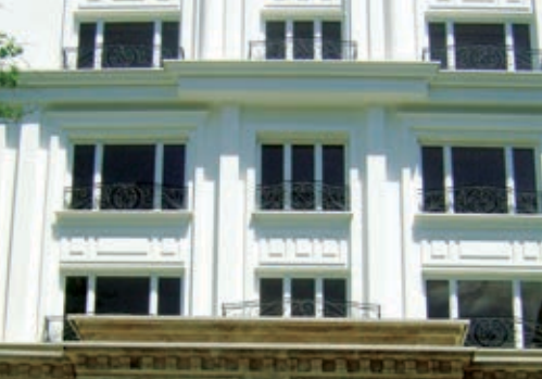
Haj Mohamadi Building Architecture: Mani Tajvar
