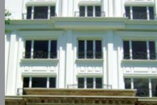
Haj Mohamadi Building Architecture: Mani Tajvar
